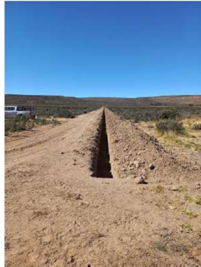
Photo 2 – Borehole 11 pipe trench to connect onto mainline
