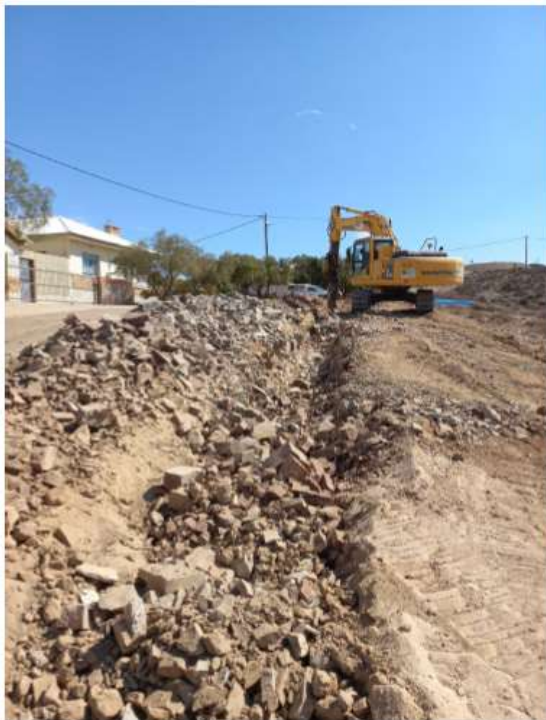
Hard rock excavations
