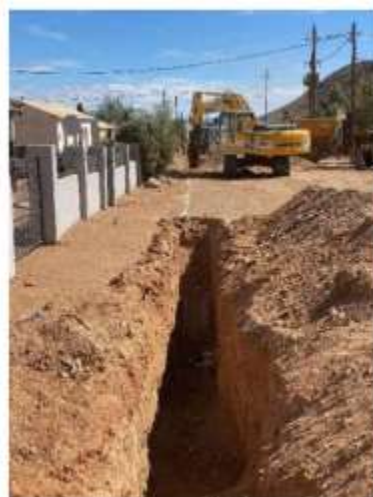
Completing last section of hard rock excavation in Spangenberg Street, Williston
