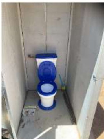
Prefabricated Toilet installation completed
