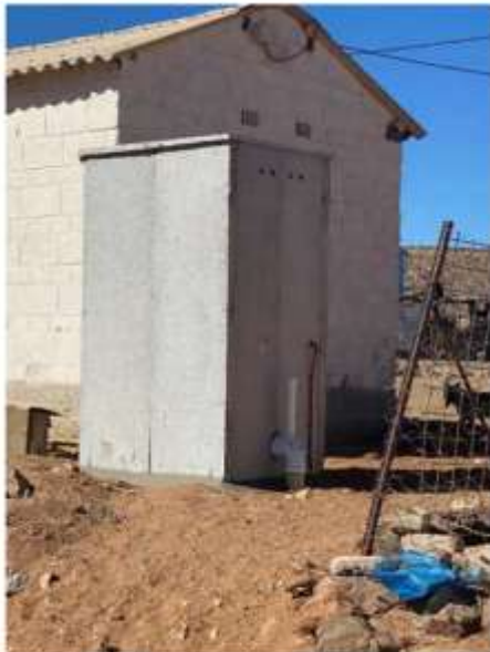
Prefabricated Toilet installation completed
