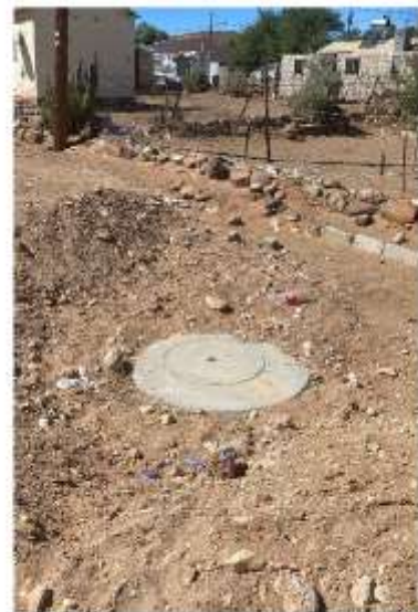
Completed sewer manhole in Vygie Street
