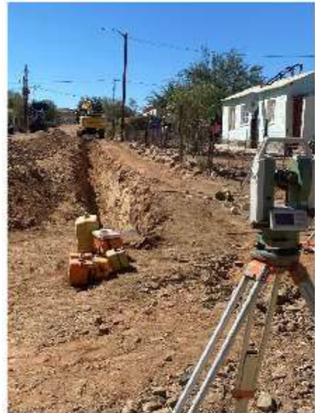
Excavation of trenches for sewer lines in Scholtz Street, Williston
