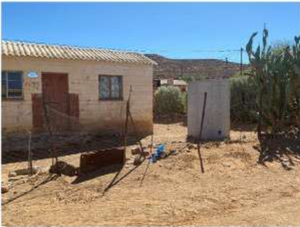
Prefabricated Toilets installed in Spangenberg Street, Williston
