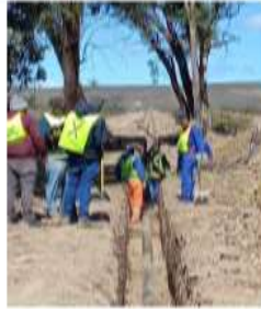
Photo 2 – Borehole 11 pipe trench to connect onto mainline
