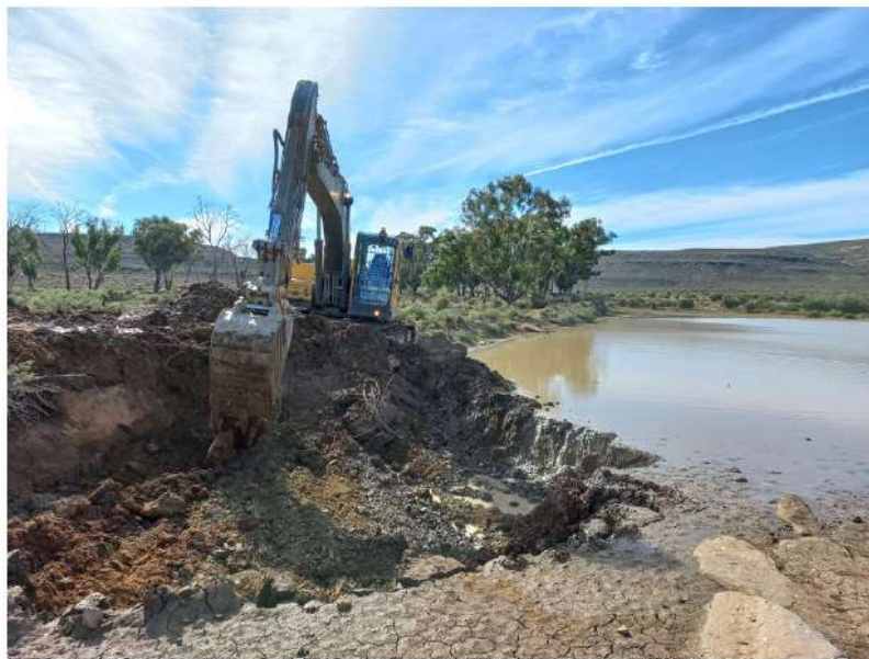
Photo 3 – Artificial Recharge structures open up at Borehole No 4
