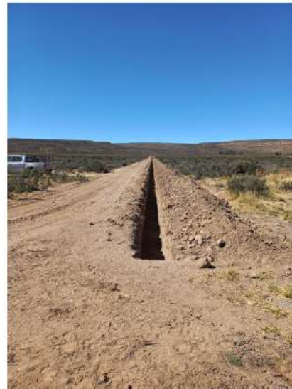
Photo 2 – Borehole 11 pipe trench to connect onto mainline
