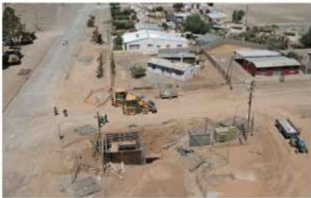
Construction of Wastewater Pump Station sump, cor. of Prins and Commercial Streets, Fraserburg
