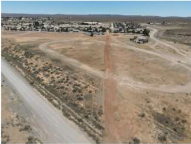
Completed and backfilled wastewater rising main to Fraserburg WWTP
