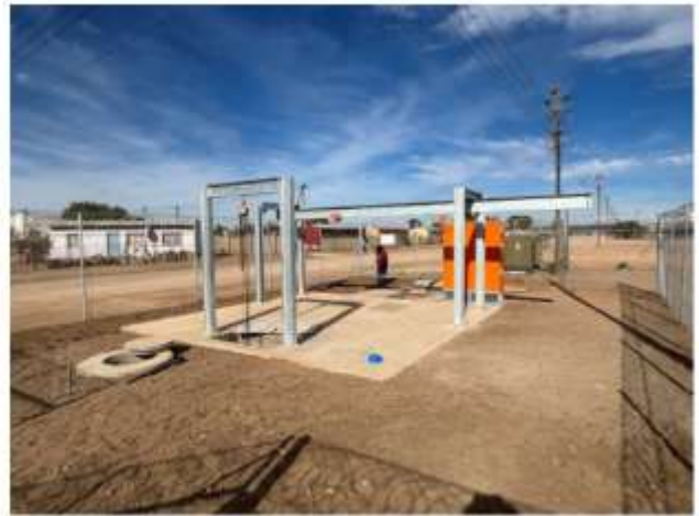
Completed Wastewater Pump Station sump
