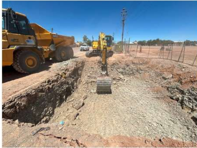
Excavation of Wastewater Pump Station sump at Fraserburg
