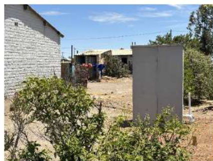
Fully assembled and connected pre-cast toilet structures
