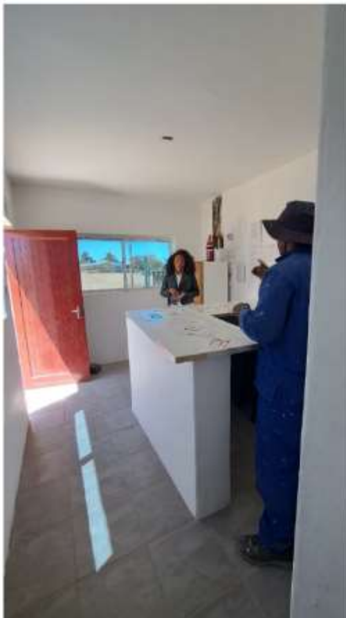
Finishing works in guardhouse
