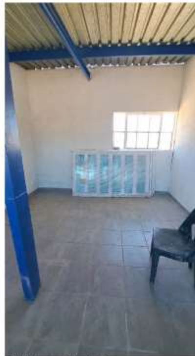
Finishing works in cloakroom
