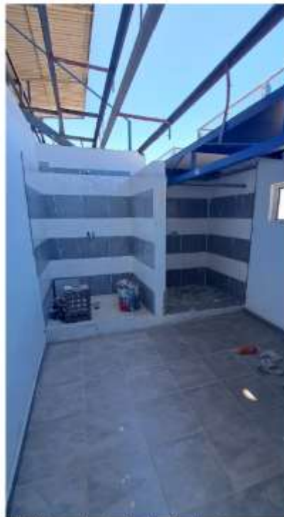
Finishing works in ablutions in cloakroom
