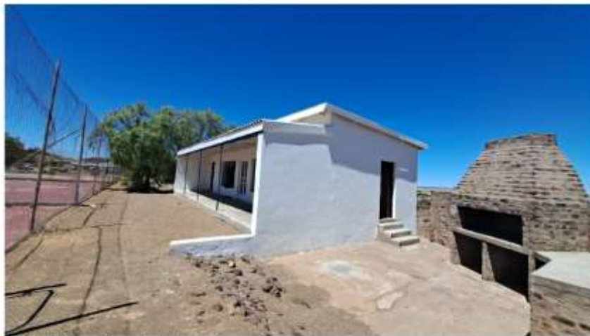
Refurbishment of tennis clubhouse
