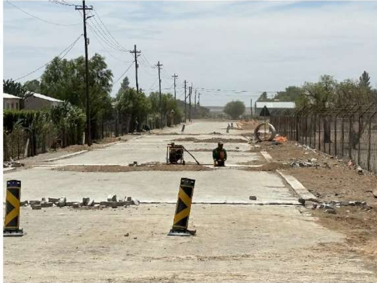
Trench excavations across paved streets for house connections
