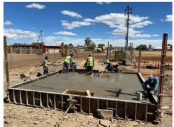
Construction of Wastewater Pump Station sump cover slab completed
