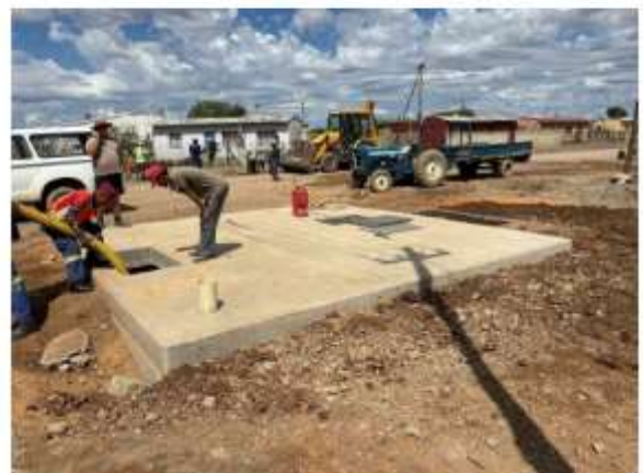
Completed Wastewater Sump for pump station
