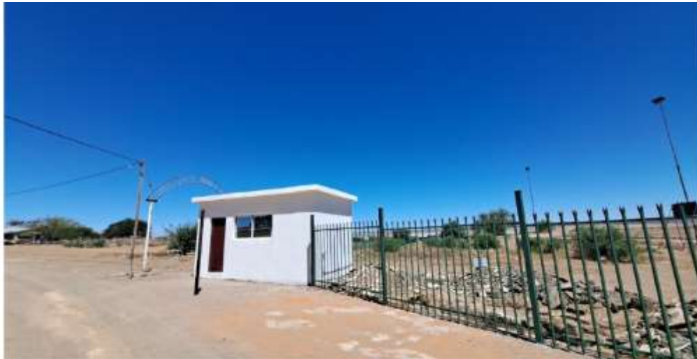
Guardhouse and perimeter fence
