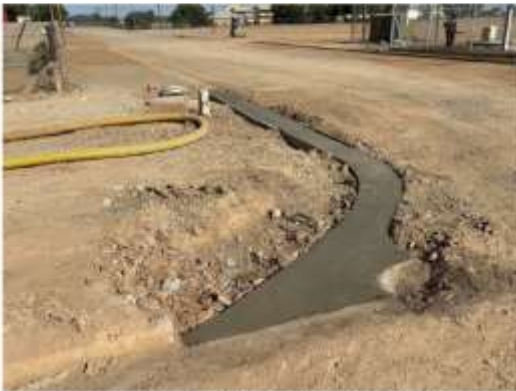
Reinstatement of kerbs and drainage gutters in Commercial Street
