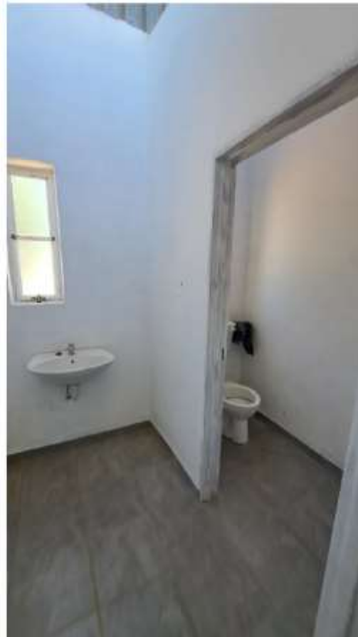
Finishing works in cloakrooms
