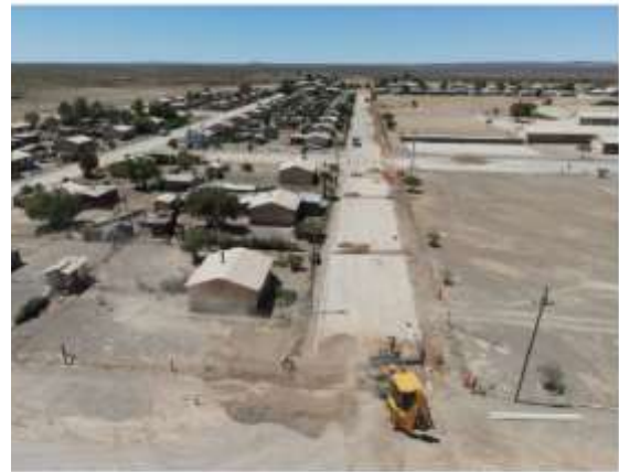
Construction of sewer lines in Blossom Street, Fraserburg
